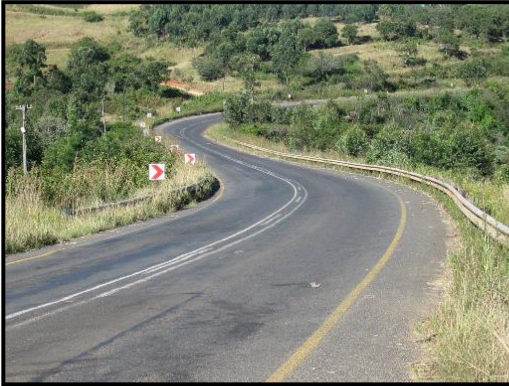
Figure 3. Photograph of the P 50-1 that is earmarked for upgrading.
